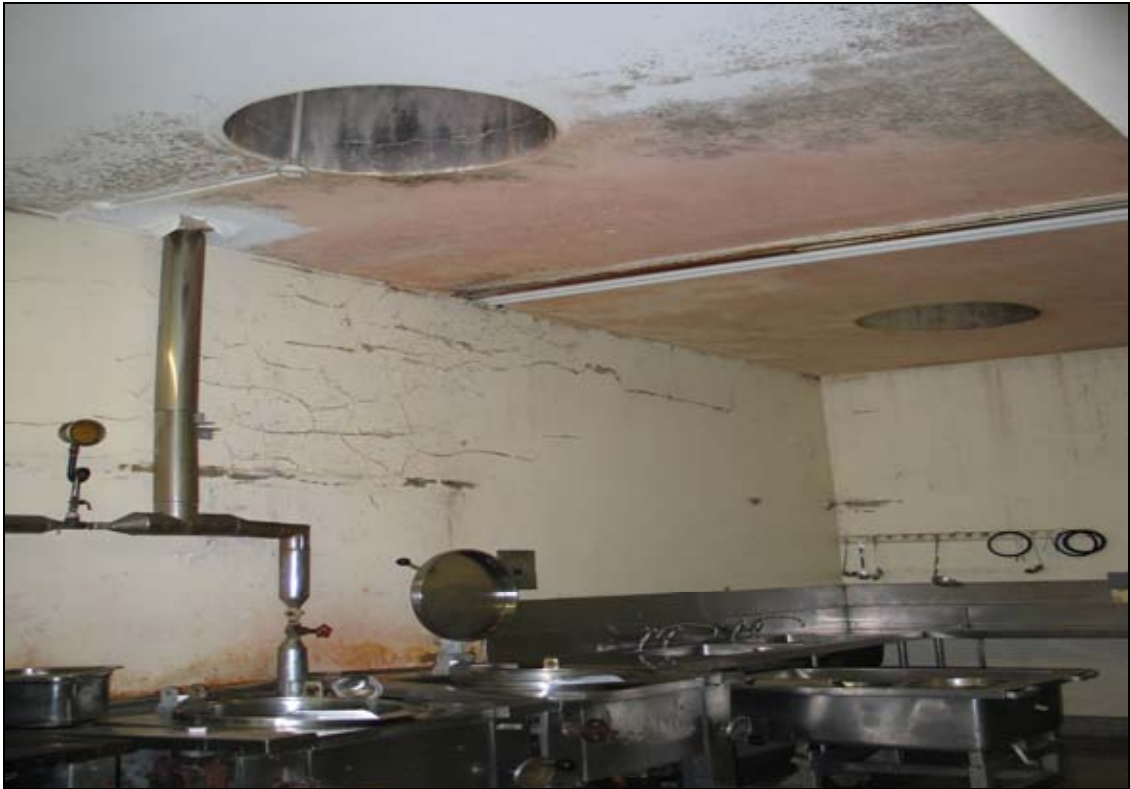
Tygerberg Hospital main kitchen: Damp and leakage noted in the kitchen and surroundings
