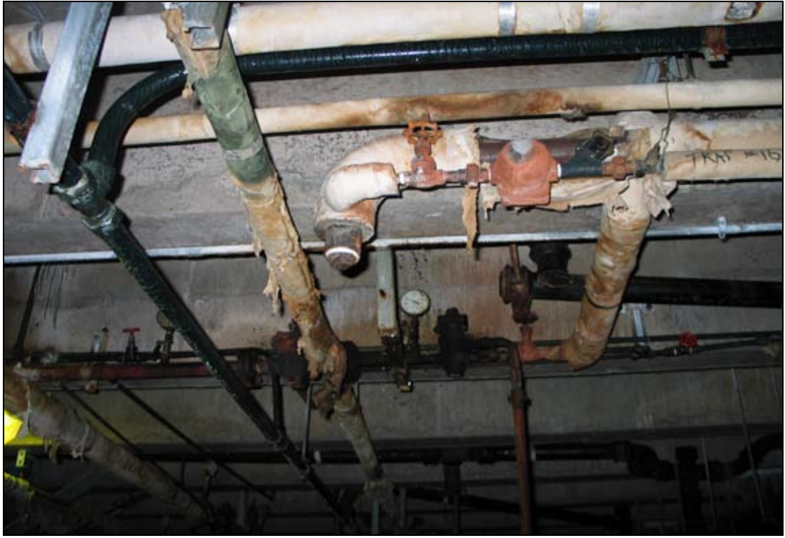
Tygerberg Hospital basement: Structural damage to pipes with water leakages
