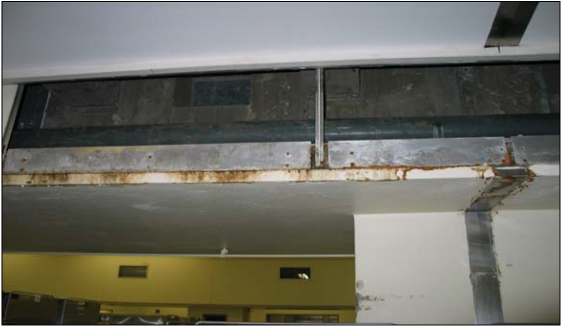
Tygerberg Hospital main kitchen: Panels missing and leakage
