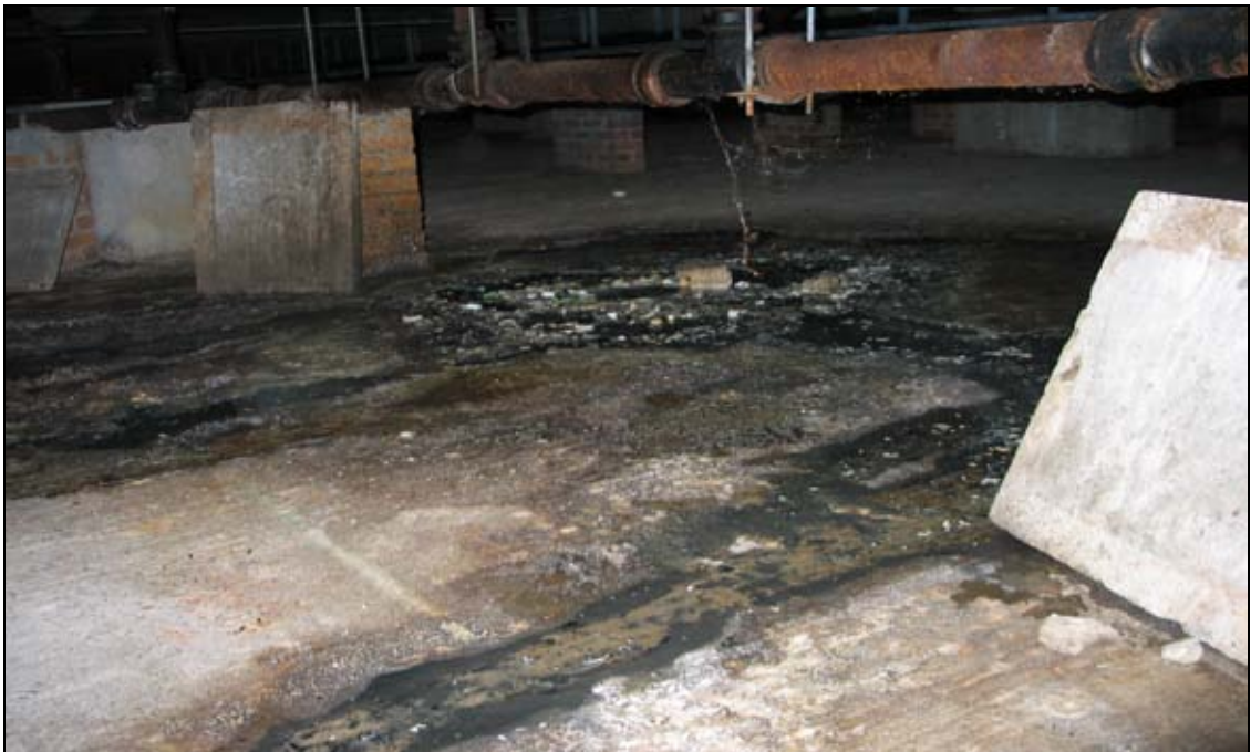
Tygerberg Hospital basement: Water leaking from dilapidated pipes and other waste from the kitchen
