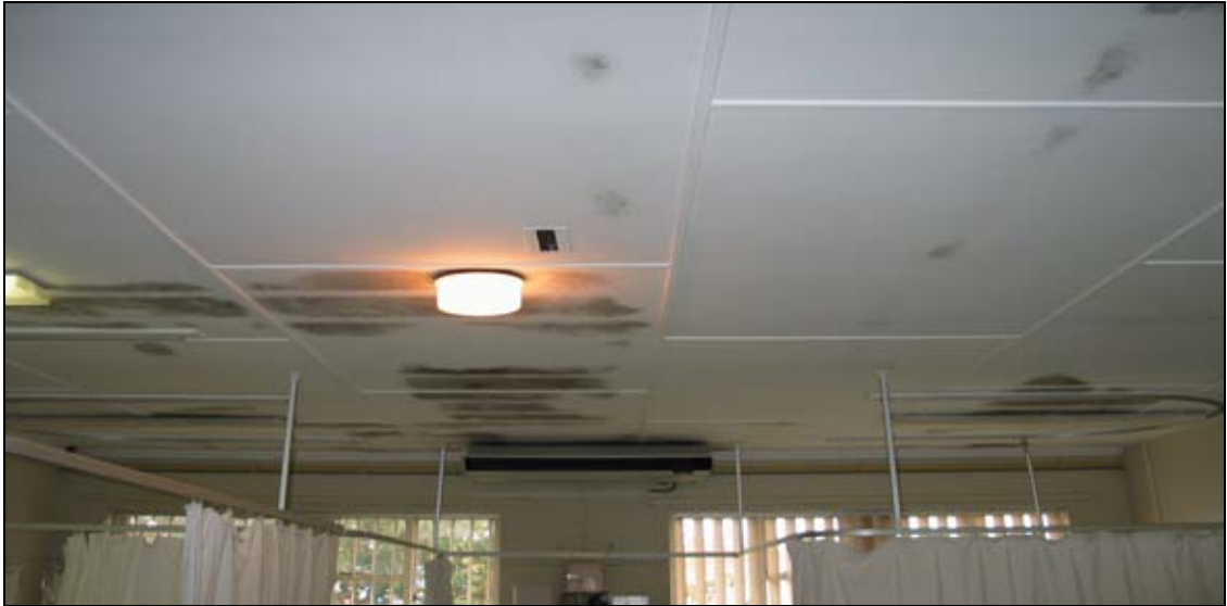
GF Jooste Hospital High Care Unit: Damp around electricity cable/light fitting
