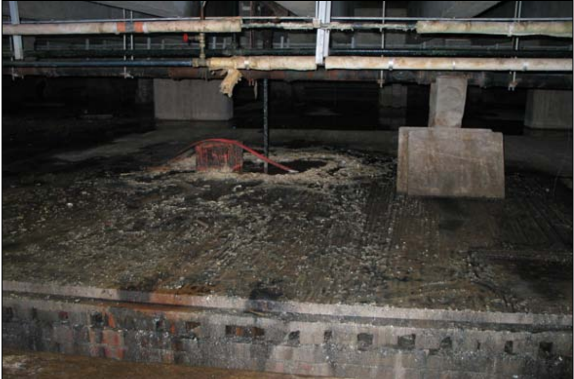
Tygerberg Hospital basement: Food and related waste leaked through the floor of the main kitchen
