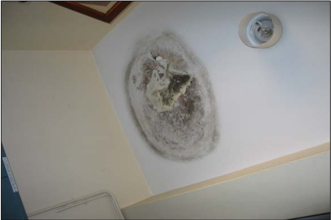
Swartland Hospital: Damp in the interior of the building close to light fitting and electricity cable
