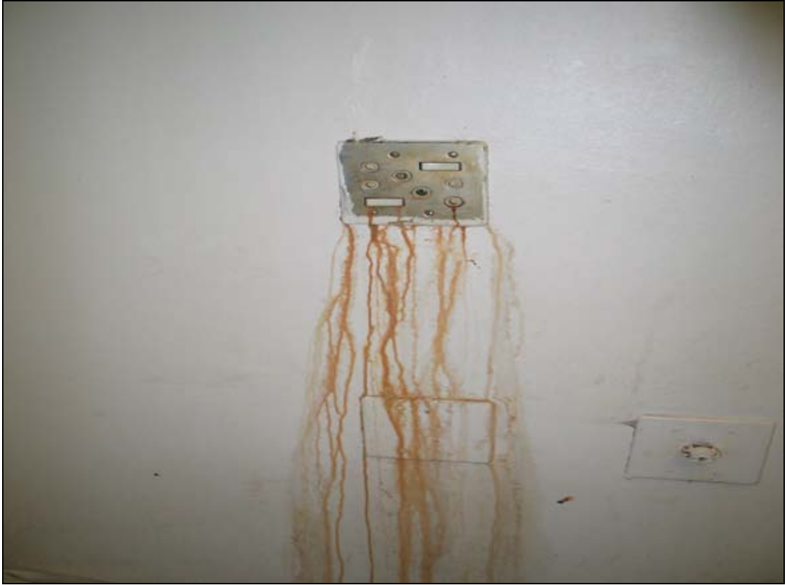
Tygerberg Hospital main kitchen: Leakage at electricity points posed safety hazards
