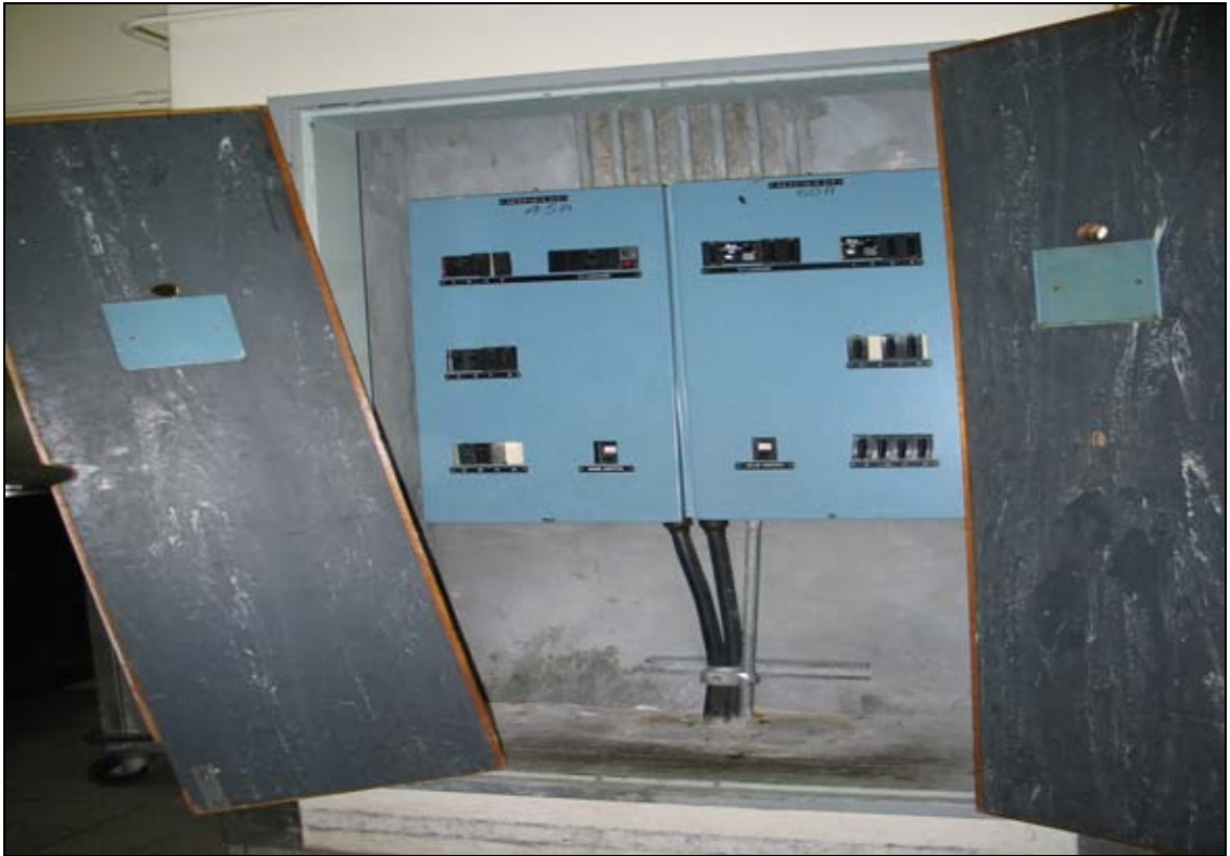
Tygerberg Hospital main kitchen: Electricity boxes open/exposed without any access control
