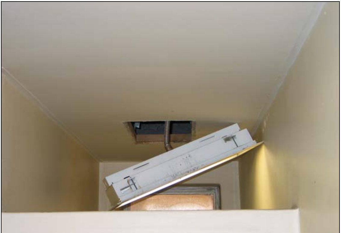
Tygerberg Hospital main kitchen: Light fittings posed injury/safety risks
