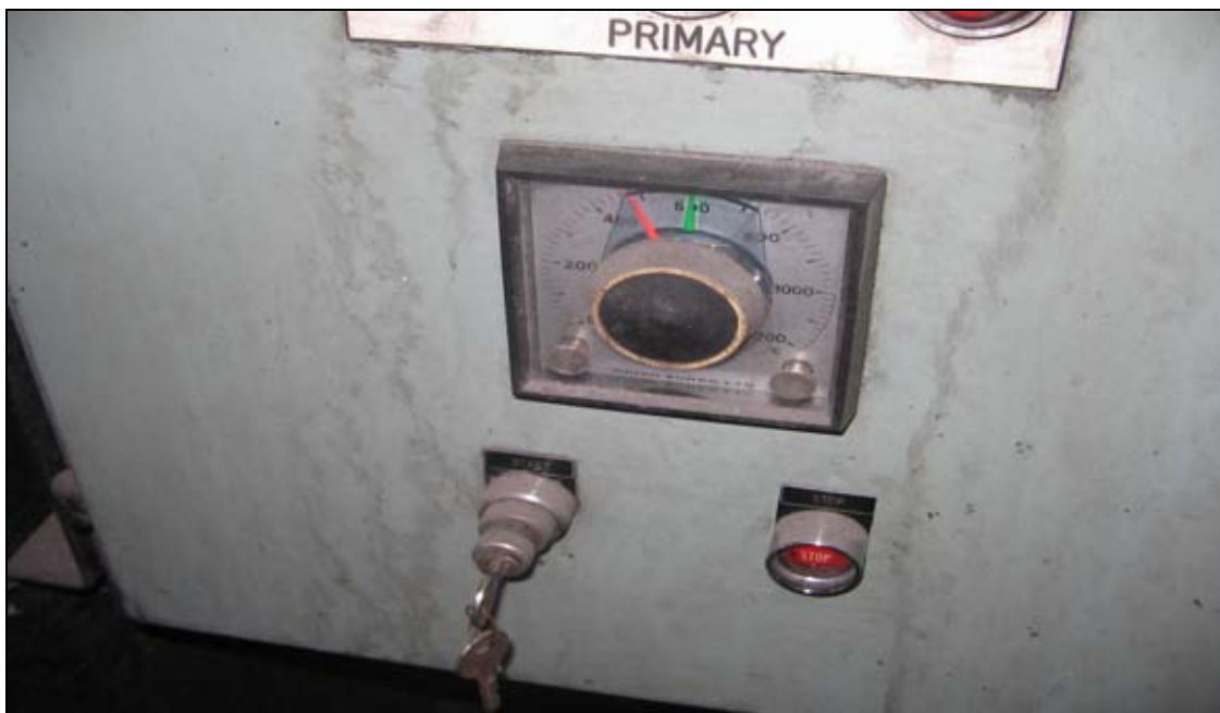
Vredendal Hospital: Incinerator set on 450 – 600 degrees
